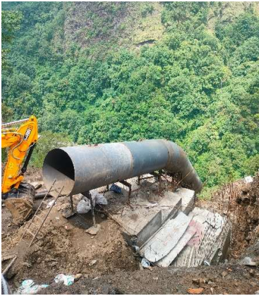
Figure 8: Anchor block construction
